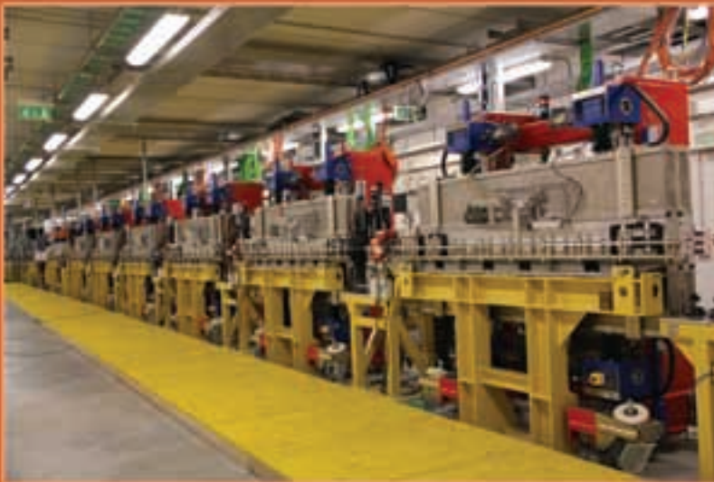
KYMA Dipole Polepiece Magnetic undulator in the FERMI@LIFE tunnel
