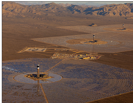
Field of dreams The Ivanpah Solar Power Facility in Nevada uses thousands of mirrors to focus sunlight onto a tank of water at the top of a tower, with the resulting steam being used to drive turbines.
