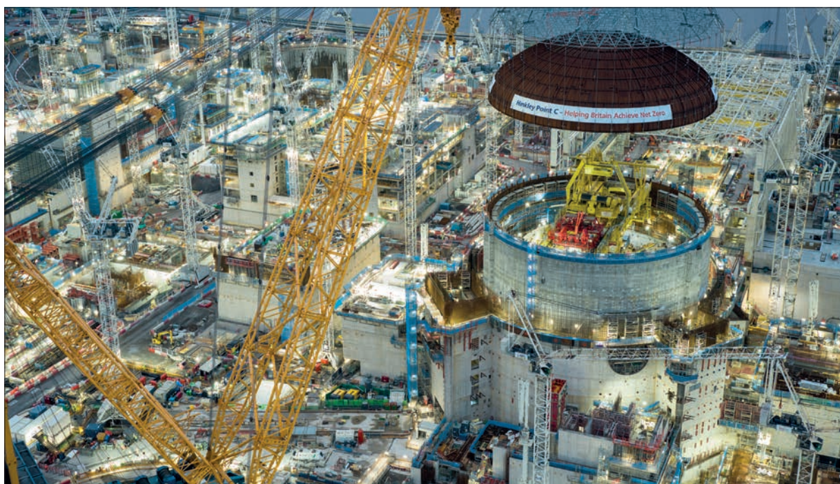
Big energy The 245-tonne domed roof has been lowered onto the first of two new reactors being built at Hinkley Point C.
