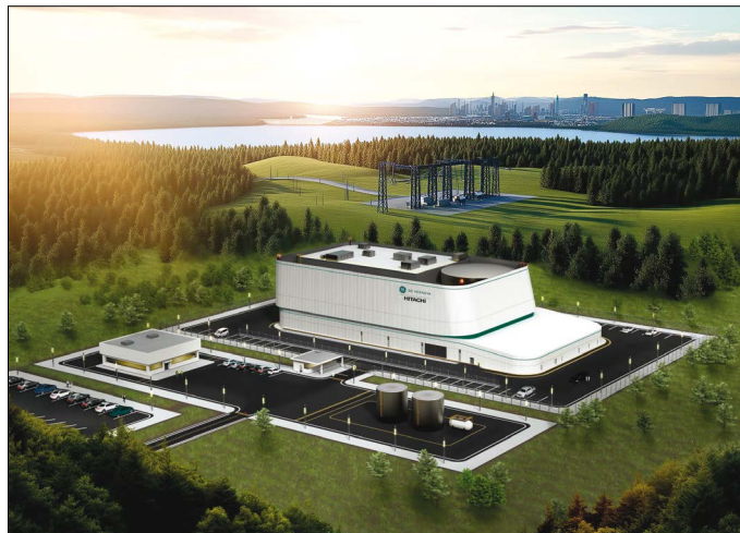
Not so small The BWRX-300 small modular reactor designed by GE Vernova Hitachi Nuclear Energy takes up around 34 acres of land. The first facility of this type is currently being built near Toronto, Canada.
